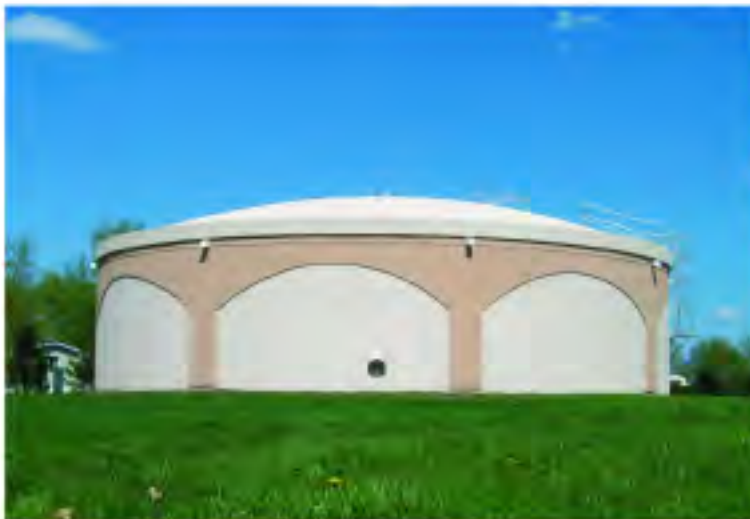
1.0 MG Natgun water tank for the City of Amboy, IL. Engineering by Felt-Graham & Associates, Freeport, IL.
